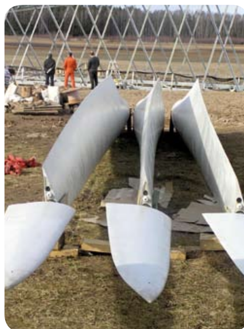
Blades of wind turbine waiting for the assembling (Photographer Gintaras Nenorta)
